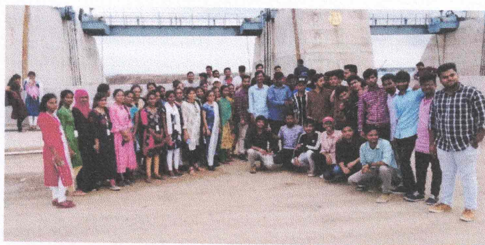
Students of Civil Engineering II year II semester, Visited KAALESHWARAM (ANNARAM, SUNDHILLA and KANNEPALLI PUMP HOUSE) PROJECT ON 26-09-2019 (AY 2019-20)
