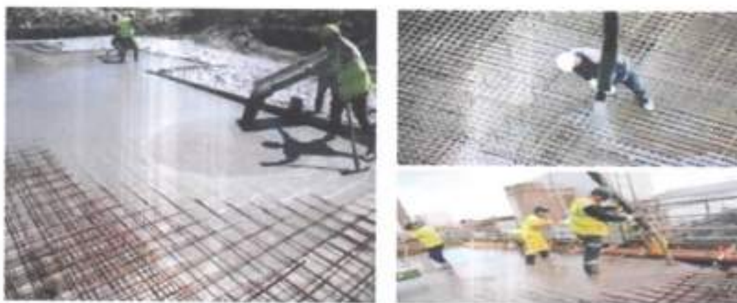
Self compacting concrete
