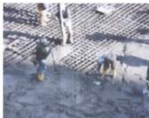
PUMPING OF CONCRETE
