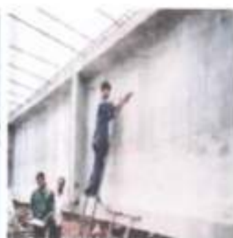
ULTRASONIC PULSE VELOCITY
